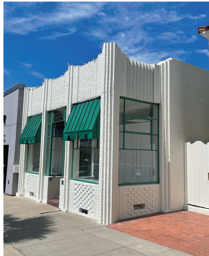
Refurbished façade to the Parker Building, where fall classes will be held
